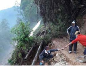
highway. The work is being carried out without proper safety mechanisms as a result of which a landslide occurred in the area yesterday. As soon as we got the message, I and a PHED team went to slide zone at Rabongla Byepass road to check the damage. We tried to restore the pipes but could not do it as even a bench
