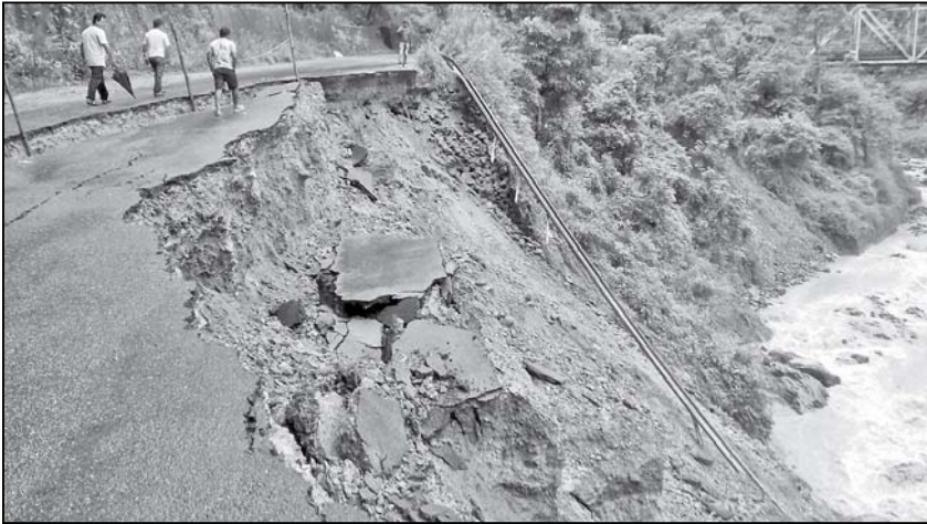
A landslide along the National Highway near Geil khola has washed away around 45 meters of road formation. However, vehicles are passing through the narrow stretch of road that still remains.
