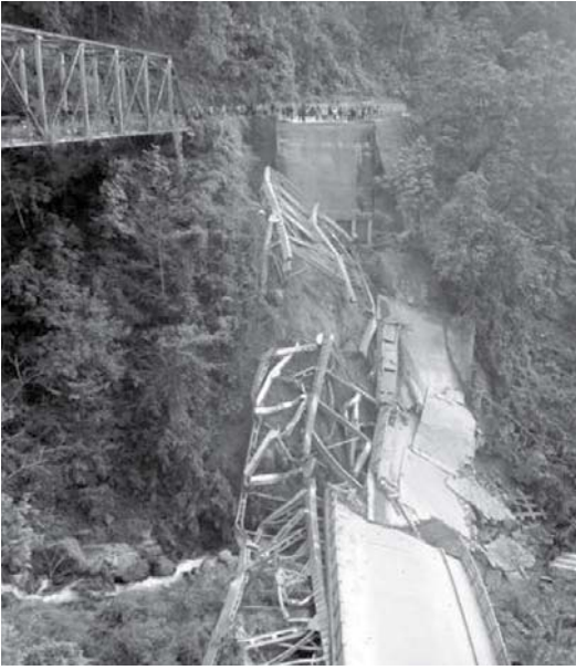
The Rangchang Bridge collapse of 19 Dec 2011. The bridge could not handle the load of a 48-wheel truck carrying 60 tonnes of load. The maximum capacity allowed on Sikkim roads at the time was 10 tonnes. Ten lives were lost in the mishap.
